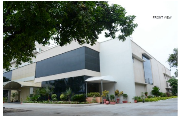
Vadodara, Gujarat, India
