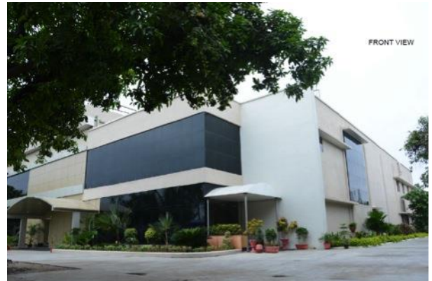
Vadodara, Gujarat, India
