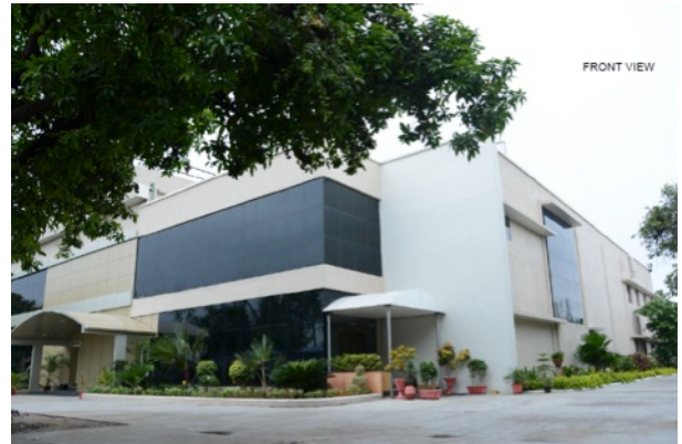
Vadodara, Gujarat, India
